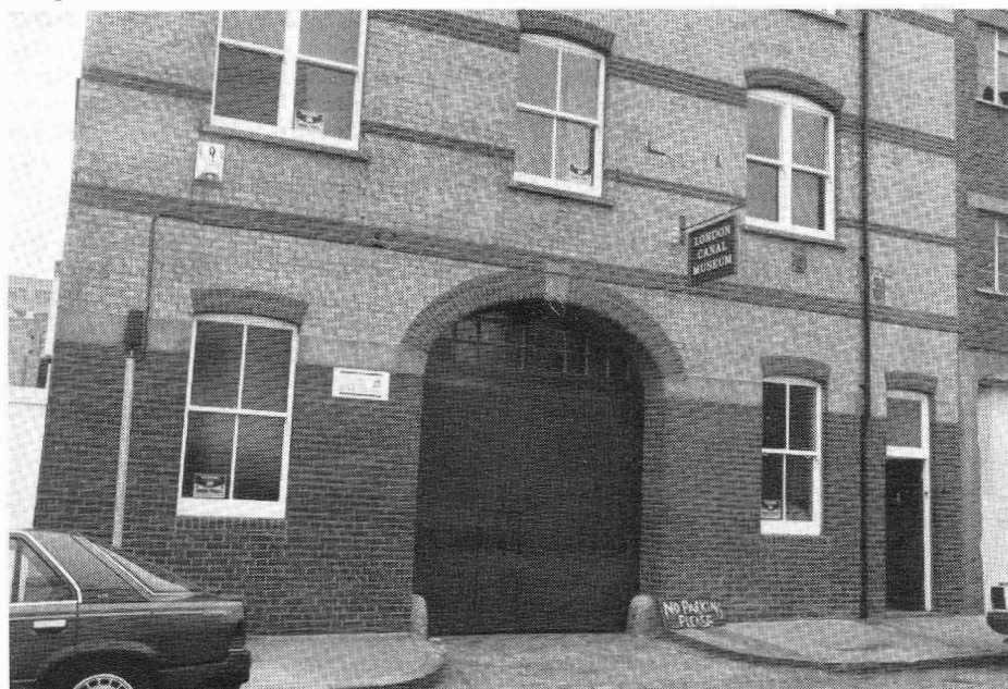
The Museum entrance in New Wharf Road
